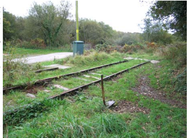
The Railway Sidings at Ponts Mill Works -
